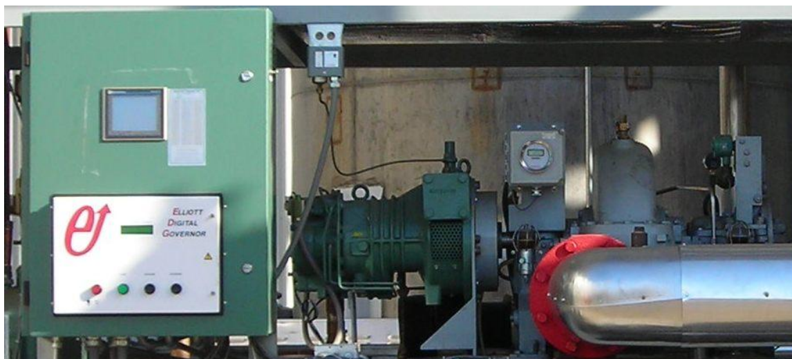
Figure 44: Steam Turbine Driven Screw Chiller
